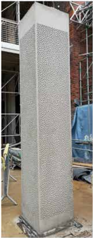
Trabecular Concrete Column Finish
